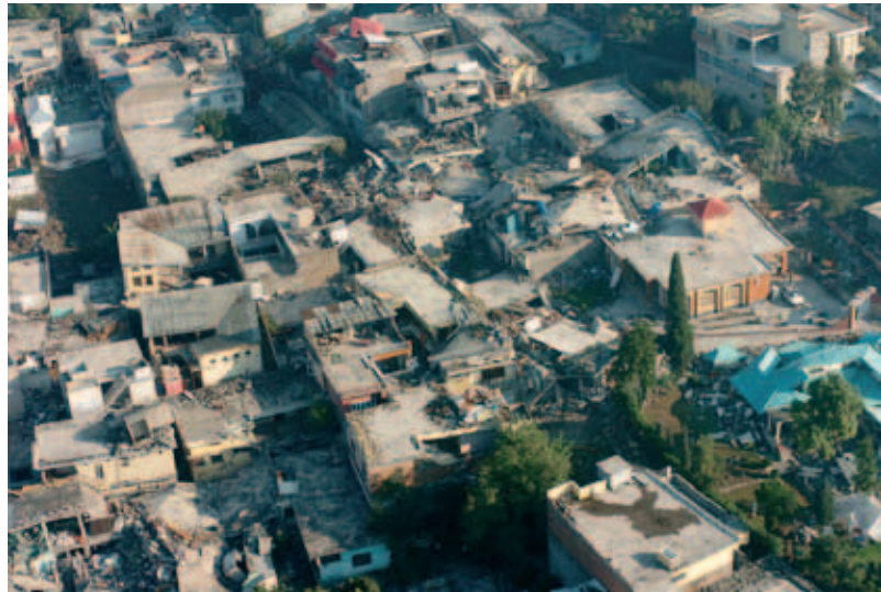
The city of Muzafarabad, Pakistan lays in ruins after the 2005 Kashmir earthquake that hit the region
